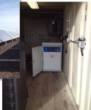
Seeo 10kWh system installed in the field with a photovoltaic array
