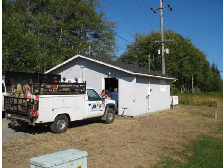
Figure 5.3. The Sekiu Pump Station Located Across the Street from Clallam PUD Facilities
