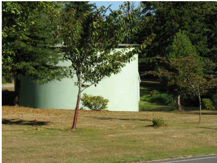
Figure 5.2. Water Reservoir Serviced by the Sekiu Pumping Station
