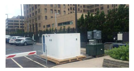
Figure 23: Repurposed 96 kWh Battery Connected to the CES PCS
