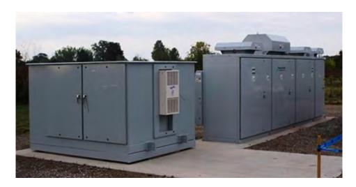
Figure 9: 500 kW Battery on the right and PCS at MCCC
