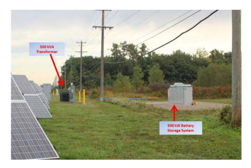
Figure 10: Ground View of 500 kW PV and Energy Storage at MCCC
