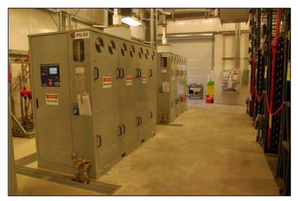
Figure 6-12 Two of the PowerCell Module PCS units (batteries at right)
