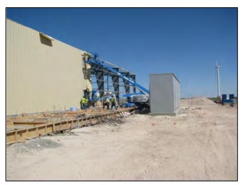
Figure 6-5 Walls along the east side of the building, with concrete forms for transformer pads in foreground and switchgear at center right (view south to north).
