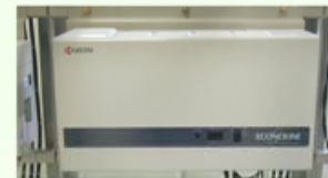
4 to 5 kW power conditioner for PV power generation
