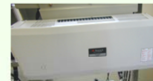
4 to 5 kW power conditioner for PV power generation
