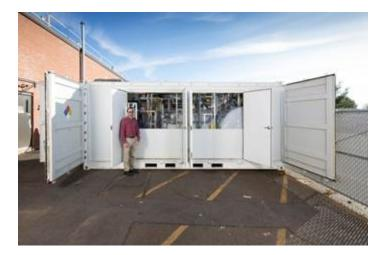
Figure 17: Vanadum redox flow battery [13].
