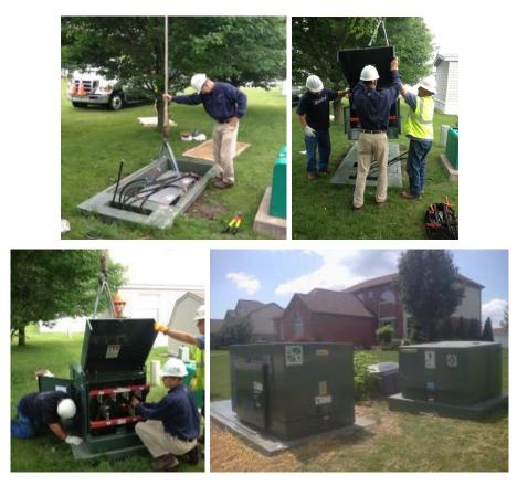
Figure 10: DTE CES system installation. In the bottom right photo, the CES is located to the left and the transformer is located on the right [9].
