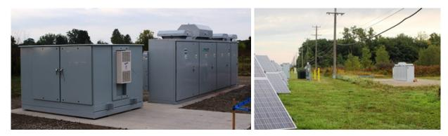
Figure 11: DTE 500 kW system collocated with a 500 kW PV [9].
