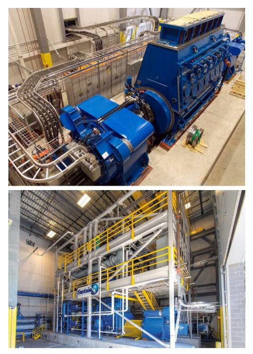
Figure 12: SustainX 1.65 MW isothermal CAES.
