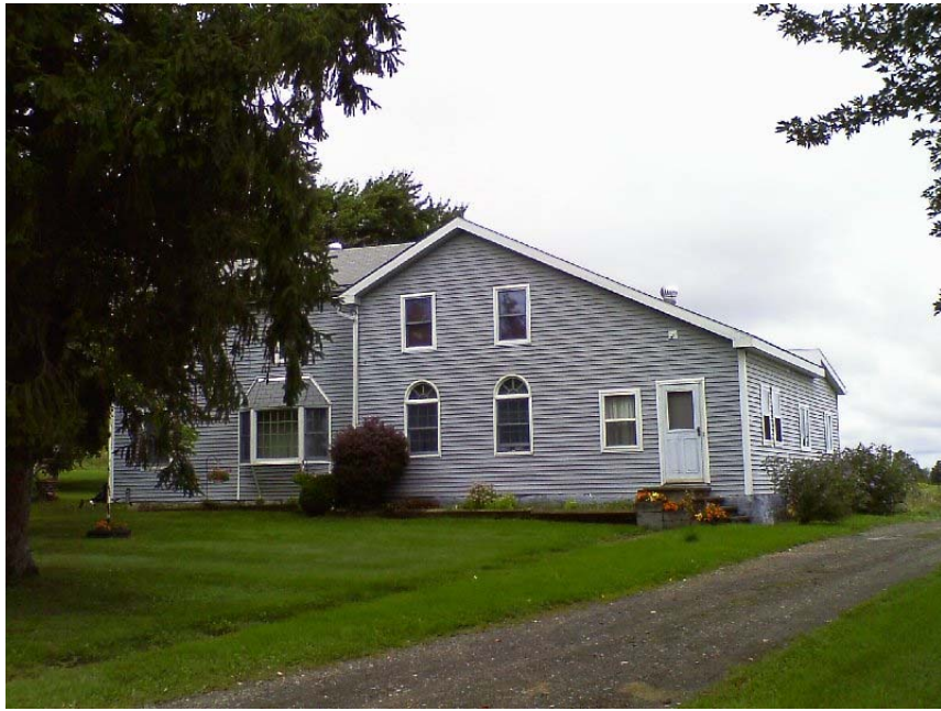
Photo Location: 3 2571 Church Road; Address given for 970.00008 (no form found) Compressed Air Energy Storage (CAES) Report ERM State Route 14A Reading, Schuylker County, NY
