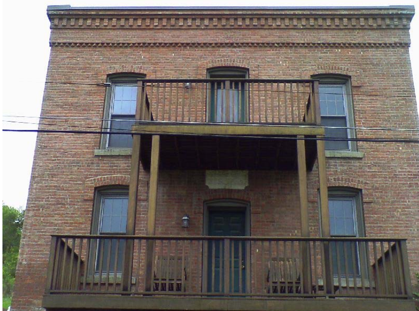
Photo Location: 4 3461 Salt Point Road; 970.00009- Seneca Lake Wine Cellar Compressed Air Energy Storage (CAES) Report ERM State Route 14A Reading, Schuylker County, NY
