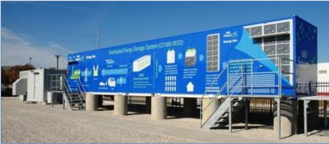
Figure 2-73: BESS Installation
