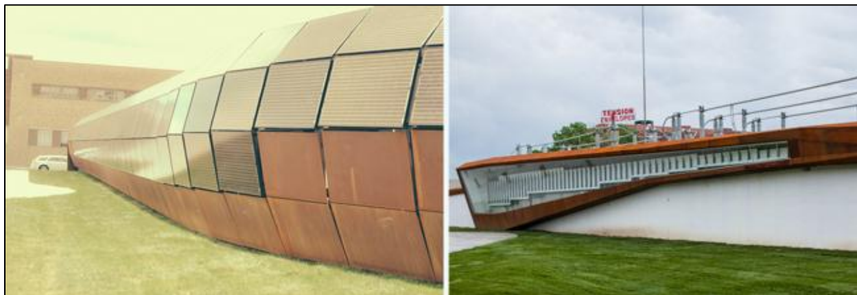
Figure 3-138: Crosstown Substation Solar Installation
