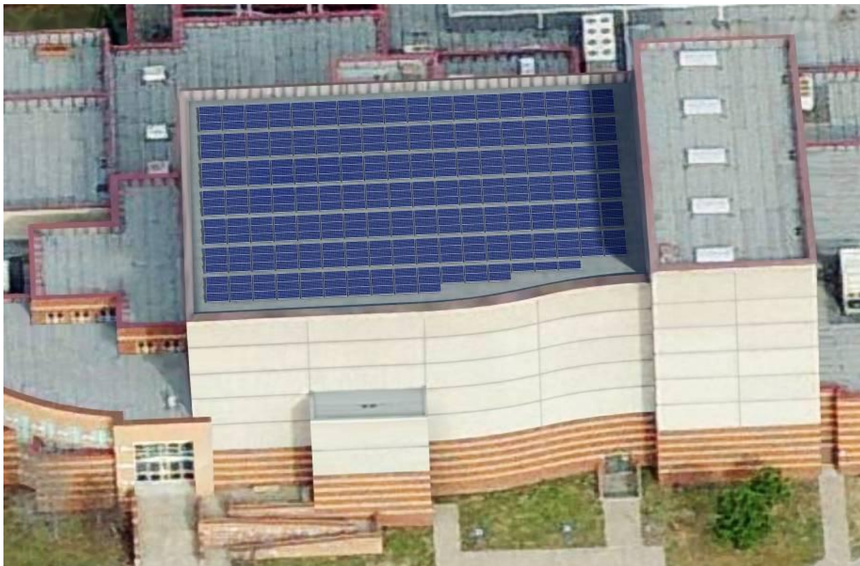
Figure 1-28: Paseo High School Rooftop Solar PV System
