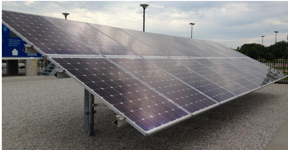
Figure 3-28: 5 kW Photovoltaic Array at SmartGrid Innovation Park
