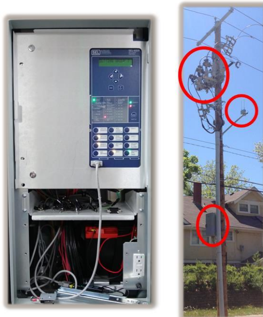
Figure 2-65: Typical Recloser Installation
