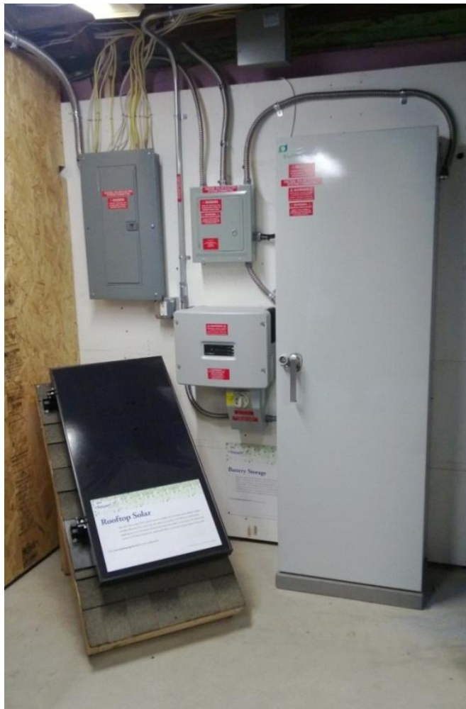
Figure 3-25: Sunverge Unit Installation at Project Living Proof Demonstration House
