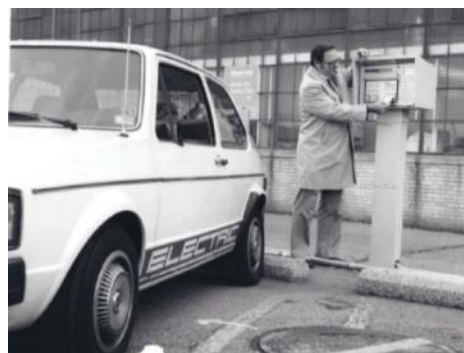
"Park & charge" credit card system, tracked energy usage and parking time for billing
