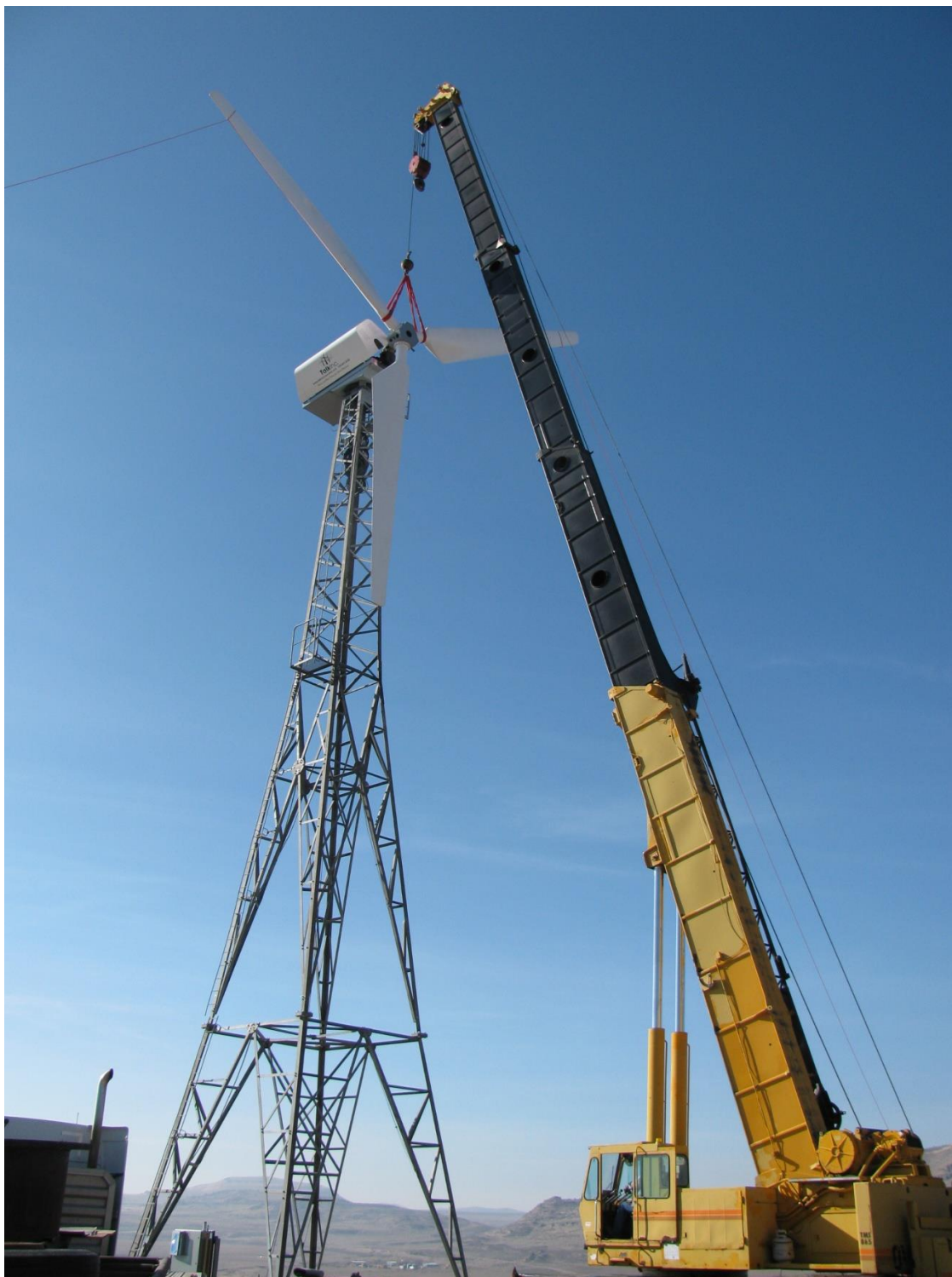
Figure 2 - Installation of 95 kW Wind Generator
